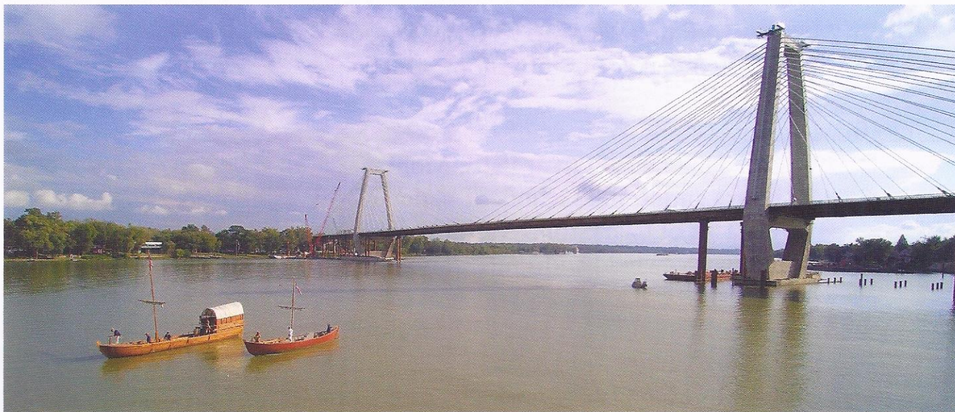
The new bridge with Lewis & Clark Discovery Expedition of St. Charles boats in foreground.
